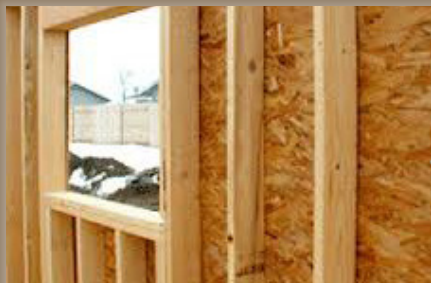
Existing Wall Structure
